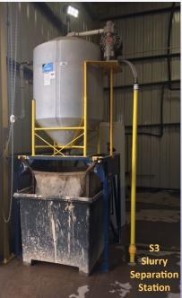
**HOW IT WORKS:** Waste concrete is washed out into the Star Hopper, where it is fed into the Concrete reclaimer. The reclaimer delivers clean sand and clean rock to separate stockpiles, and cement slurry leaves the reclaimer via the drain, where it is collected in the slurry collection pit.
